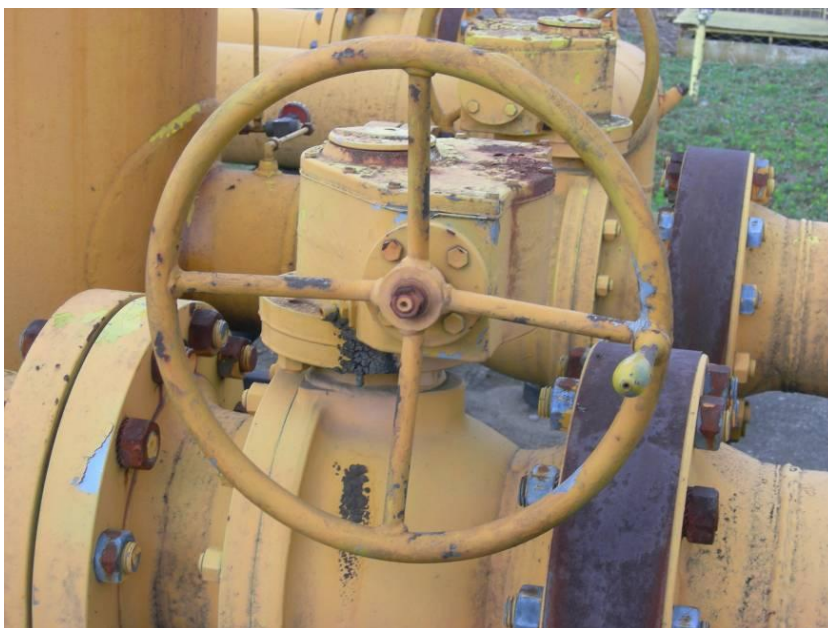
Figure 3 Distribution network valve
