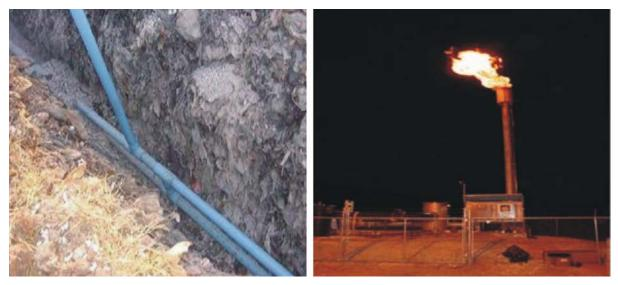
Figure 4. LFG collection and flaring system
